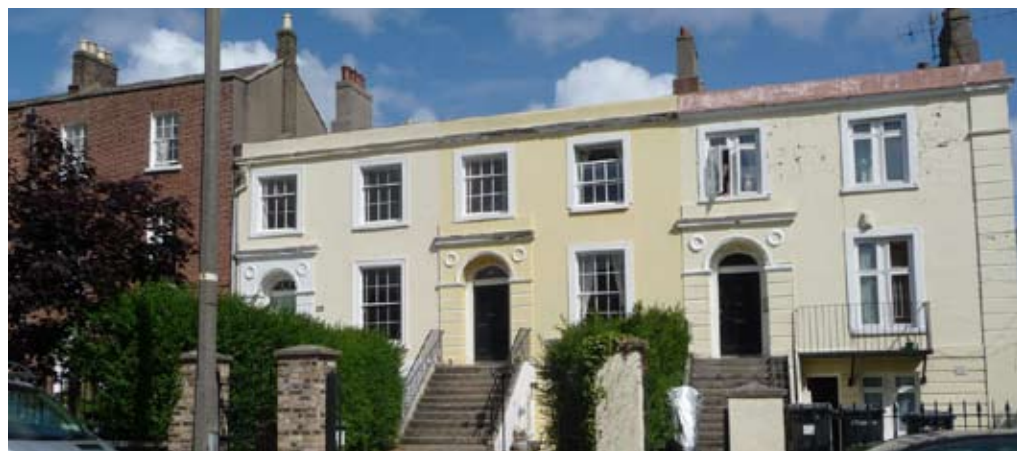
Houses built in the Regency Style on the Rathmines Side. Note the wrought Iron balconies.
